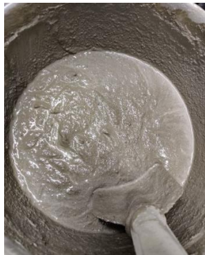
Figure 13: Mortar Mix for Beams
