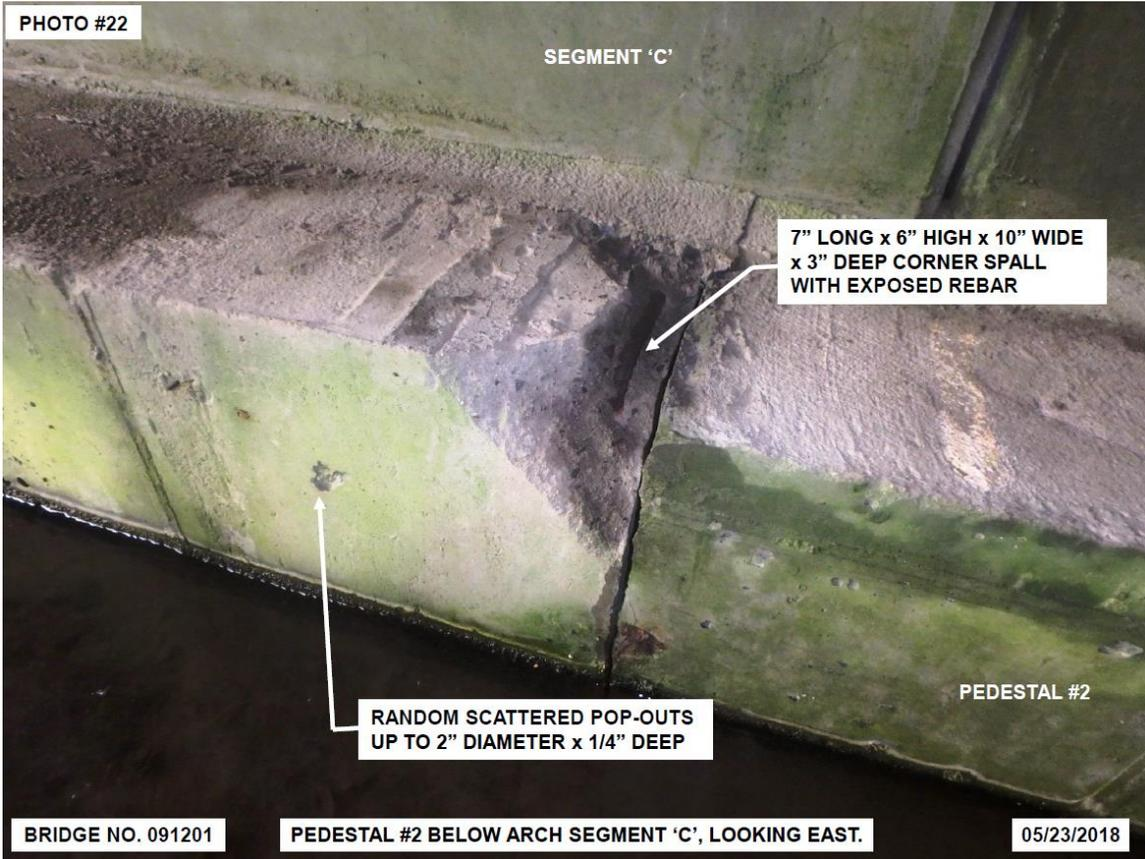
**Figure 84: Arch IV Pedestal 2C, Conventional Inspection Report (RIDOT, 2018b)**
