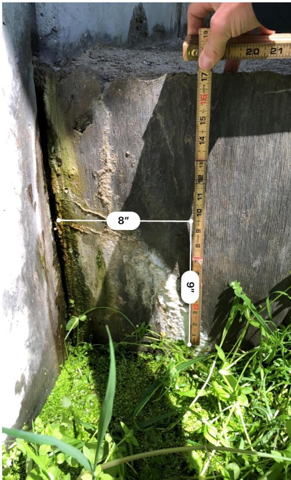
Figure 78: Arch IV Pedestal 1S, ID 2020 215-1120, Quantified Extent Height (own photo)
