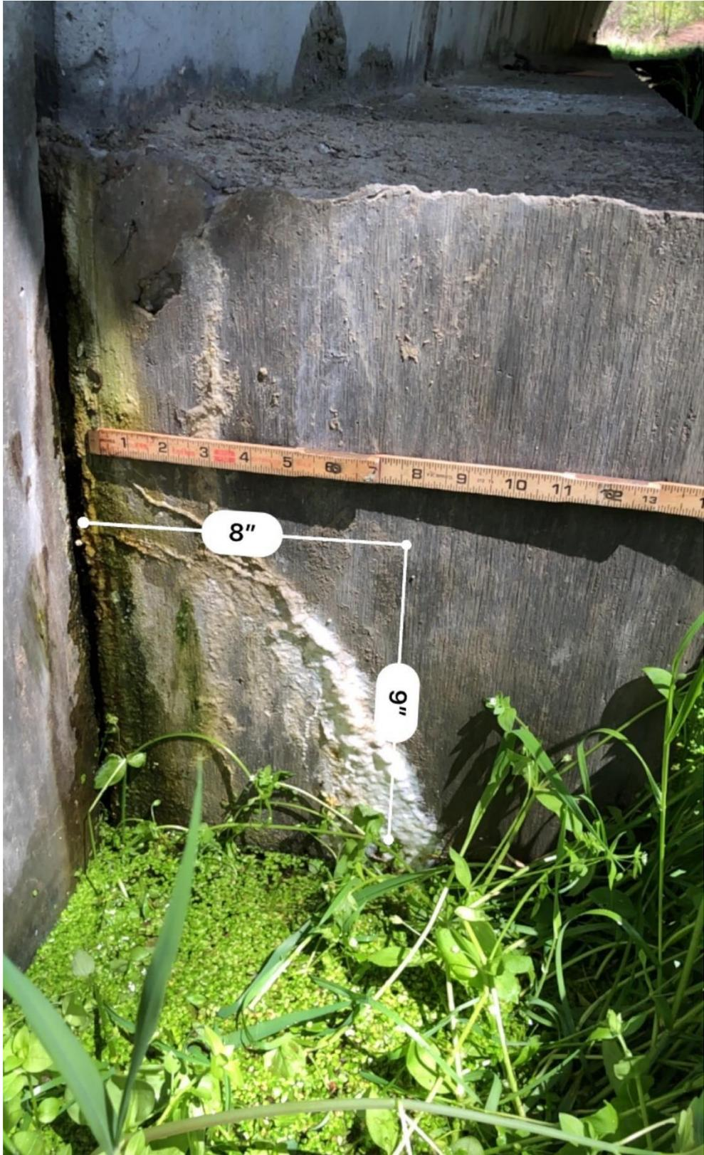
Figure 77: Arch IV Pedestal 1S, ID 2020 215-1120 Quantified Extent Width (own photo)
