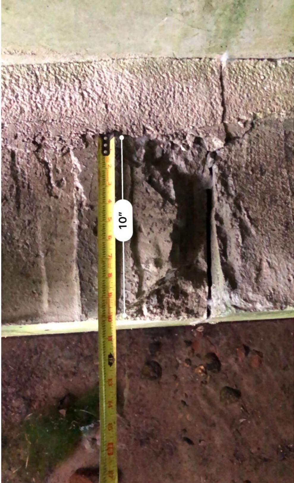
**Figure 87: Arch IV Pedestal 2C, ID 2021 215-1080, Defect Width (own photo)**
