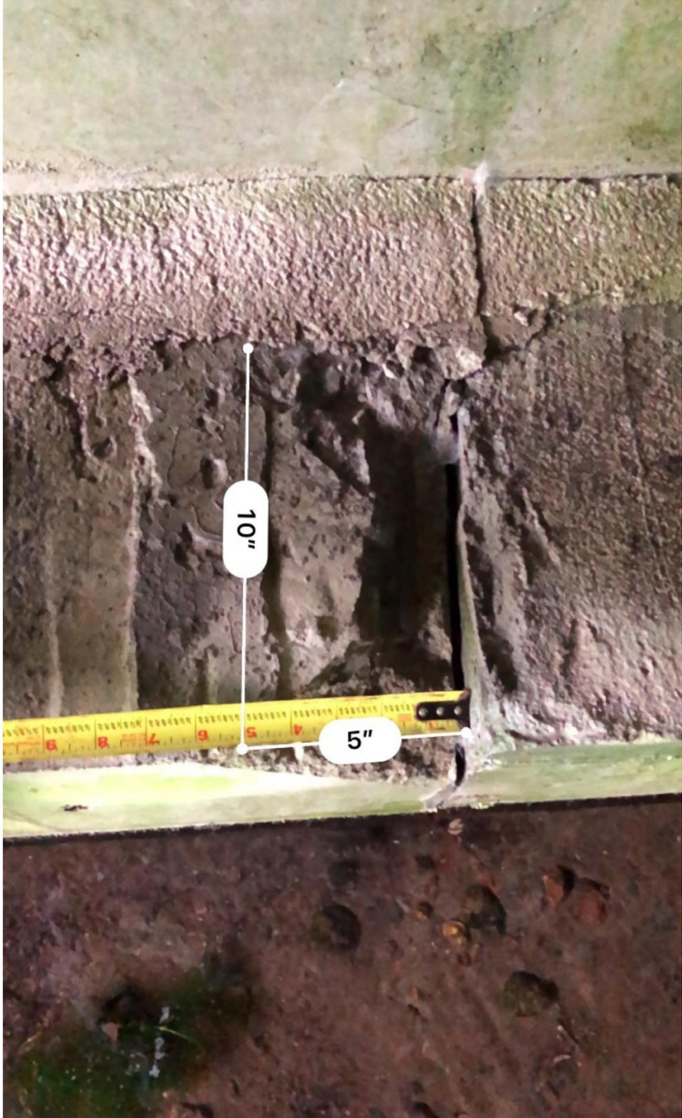
Figure 86: Arch IV Pedestal 2C, ID: 2021 215-1090, Defect Length (own photo)
