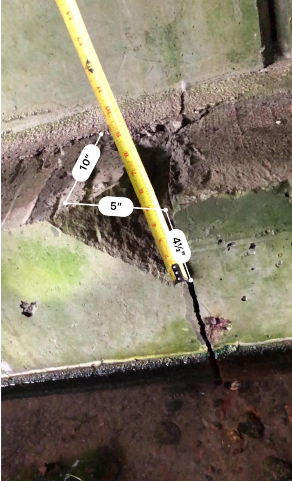
Figure 88: Arch IV Pedestal 2C, ID 2021 215-1090, Defect Height (own photo)
