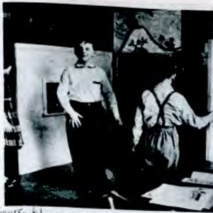
Figure 61 ERECTING FRAMEWORK for the pet shop was boys' job. Proud of his part in it is Kevin McBride, center.
