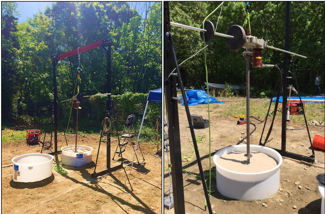
Figure 7 – Photographs of the test site setup with driver and anchor attached.
