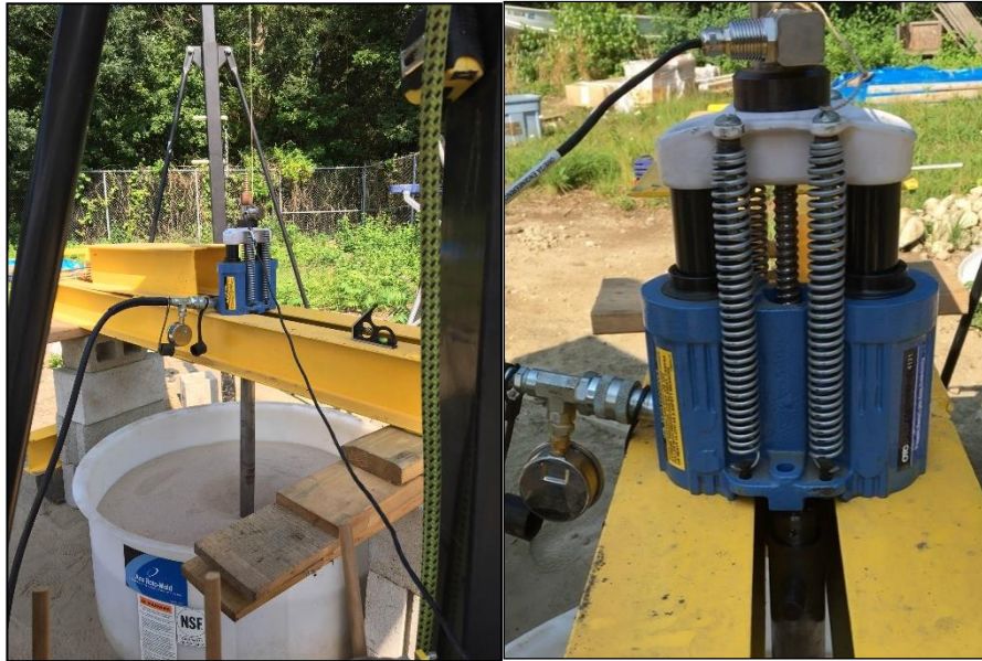
Figure 20 – Photograph of a pullout performed by pneumatic jack system
