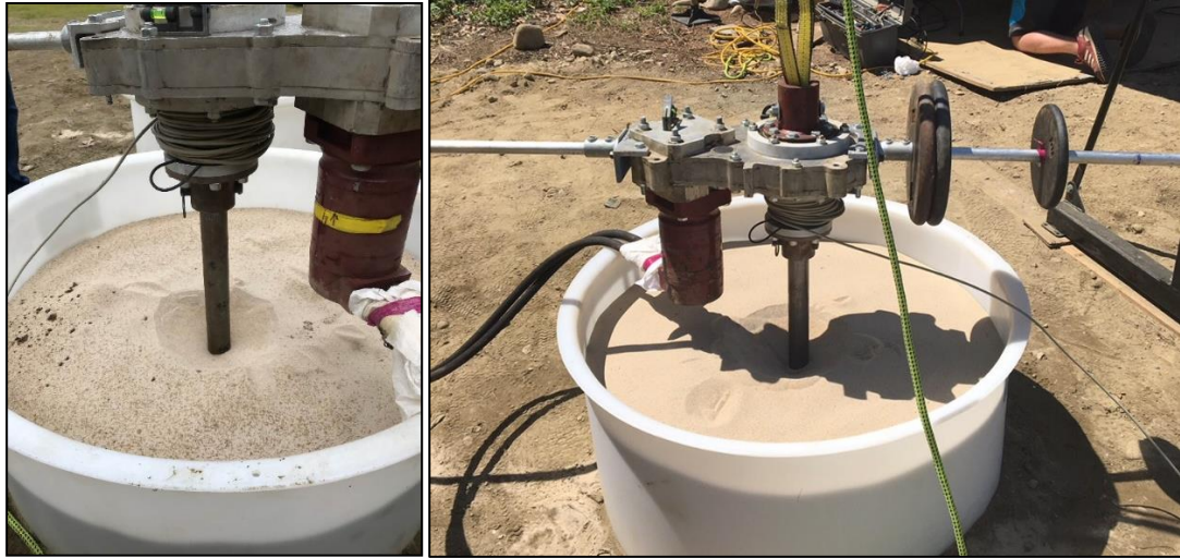
Figure 19 – Photograph of the driver and a fully installed anchor in loose sand
