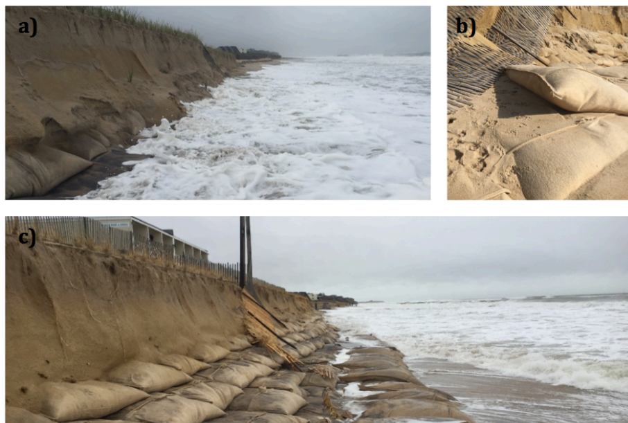
Figure 2.3 Post construction surveys and monitoring. a) Photo taken in September 6, 2016 during TS Hermine. b) Photo taken in September 9, 2016 after TS Hermine. c) Photo taken during January 24, 2017 Nor'easter storm. (Photo credit: Brian Maggi)
