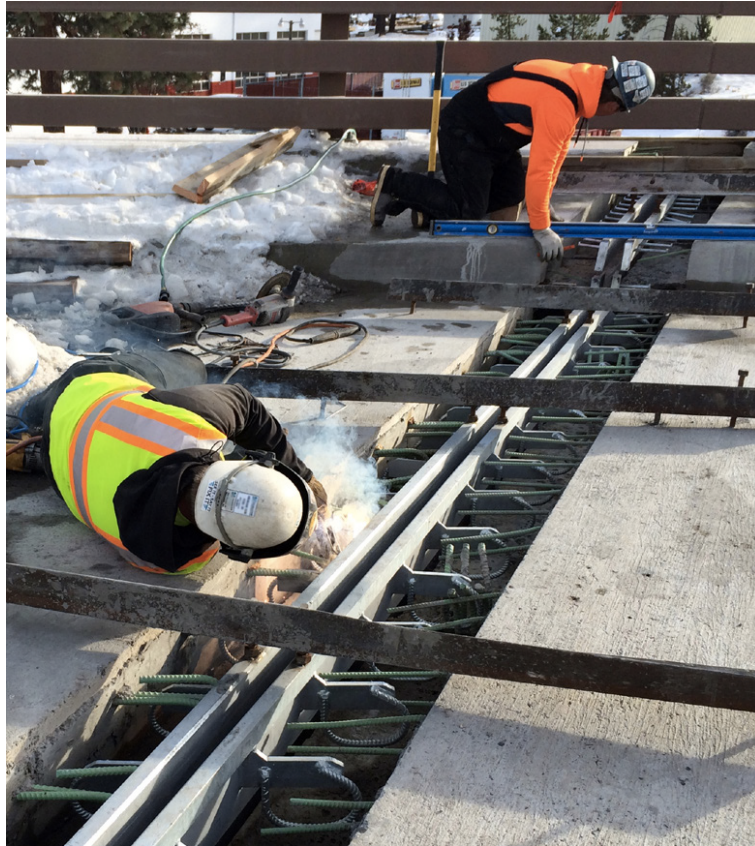
Picture 10: Joint replacement (FHWA 2018d)
