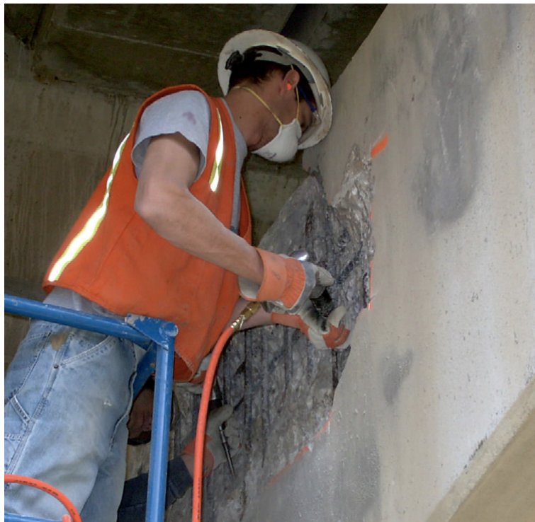
Picture 9: Substructure repair (FHWA 2018d)
