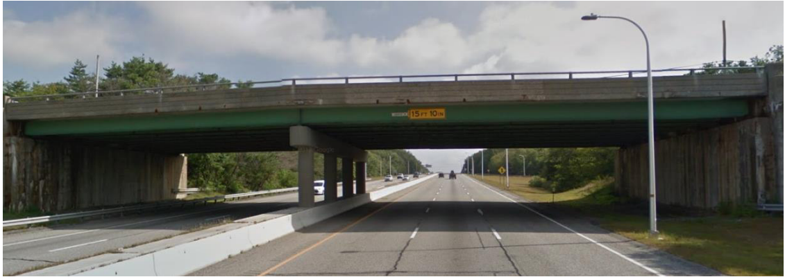
Figure 11 - Canonchet Bridge on I-95 northbound (Google Maps 2017)
