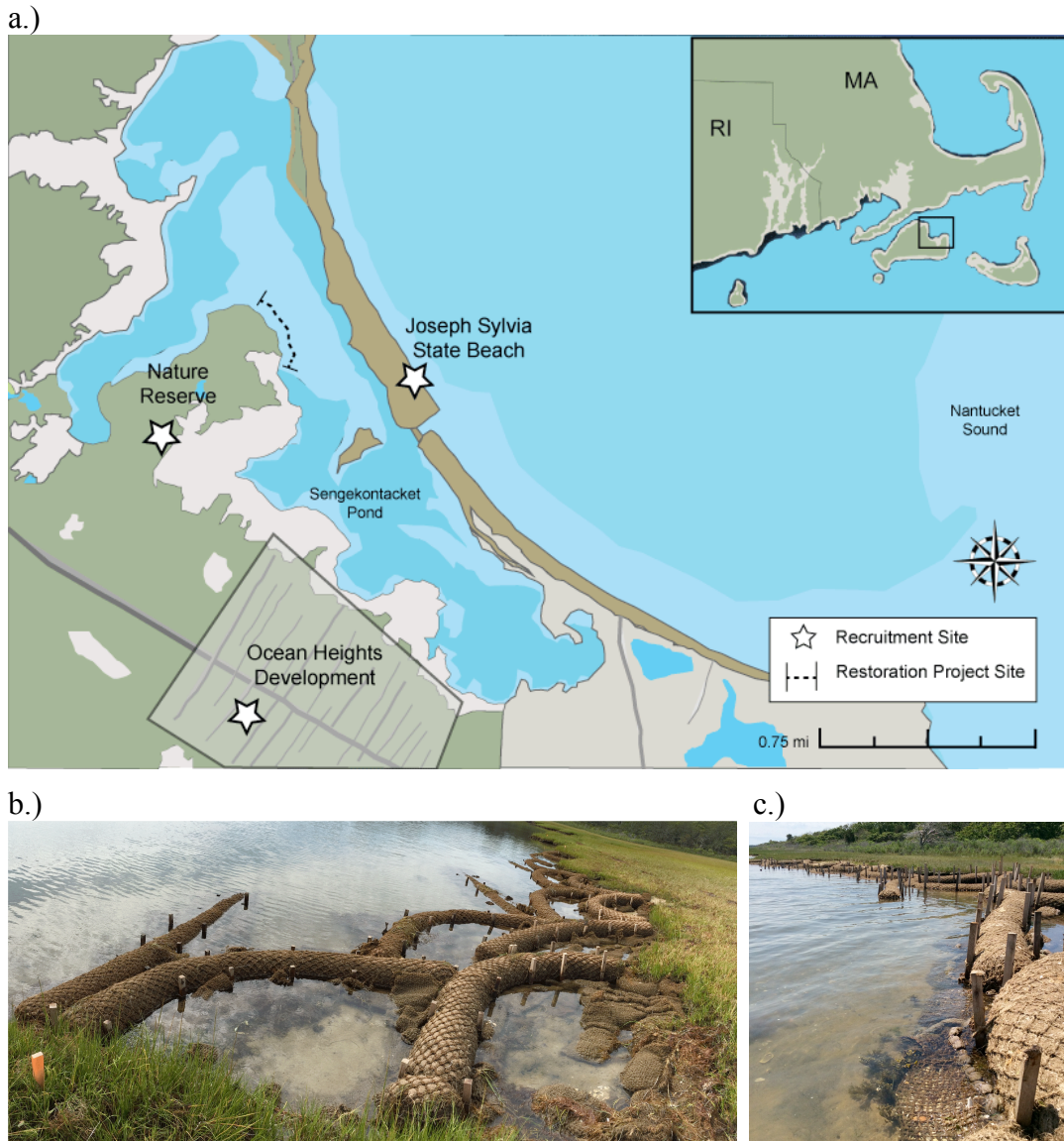
Figure 1. Study site including a.) locations of interview recruitment sites relative to the living shoreline restoration project site, b.) living shoreline restoration project, and c.) detail of living shoreline design using coconut fiber logs and bags of oyster shell as a biodegradable shoreline stabilization and salt marsh habitat facilitation structure.
