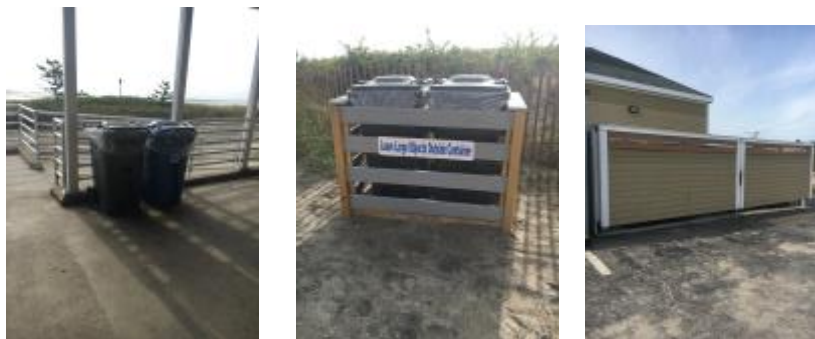
Figure B. From left to right: trash and recycling totes on the pavilion, trash and recycling totes in a corral on the beach, and enclosed dumpster all located at Narragansett Town Beach.
