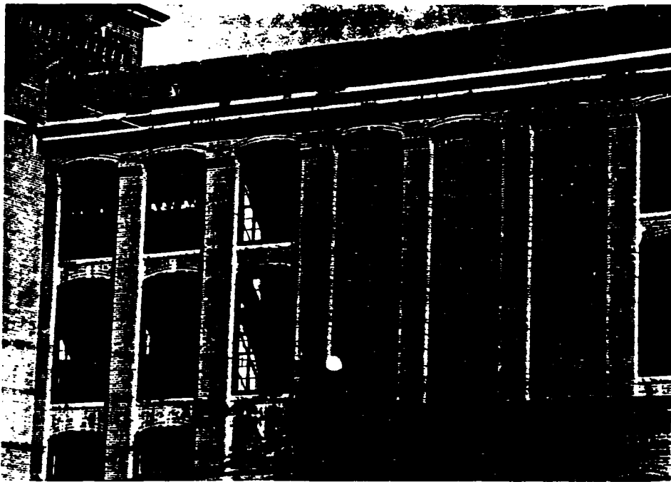
Brick-pier construction
