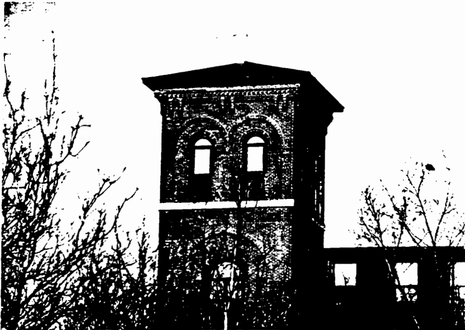
Peaked roof tower
