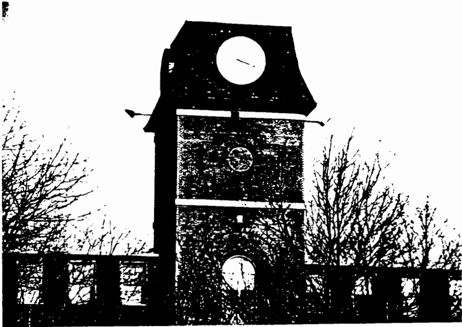
Mansard roof tower
