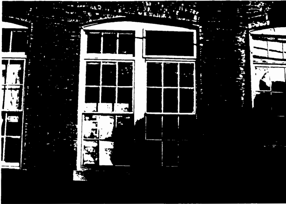
Paired windows with transom
