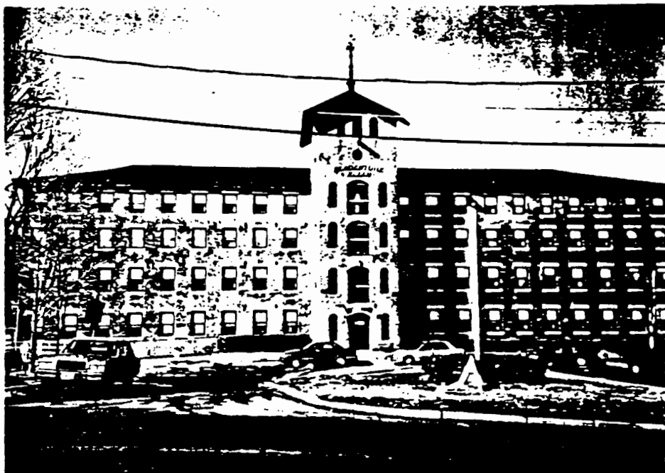
Valley Falls Company Mill
