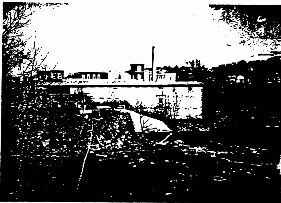
Falls Yarn Mill (Proximity to River)
