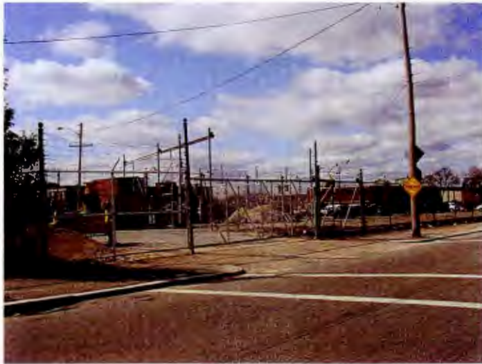
Narragansett Electric next to Sackett Street Park
