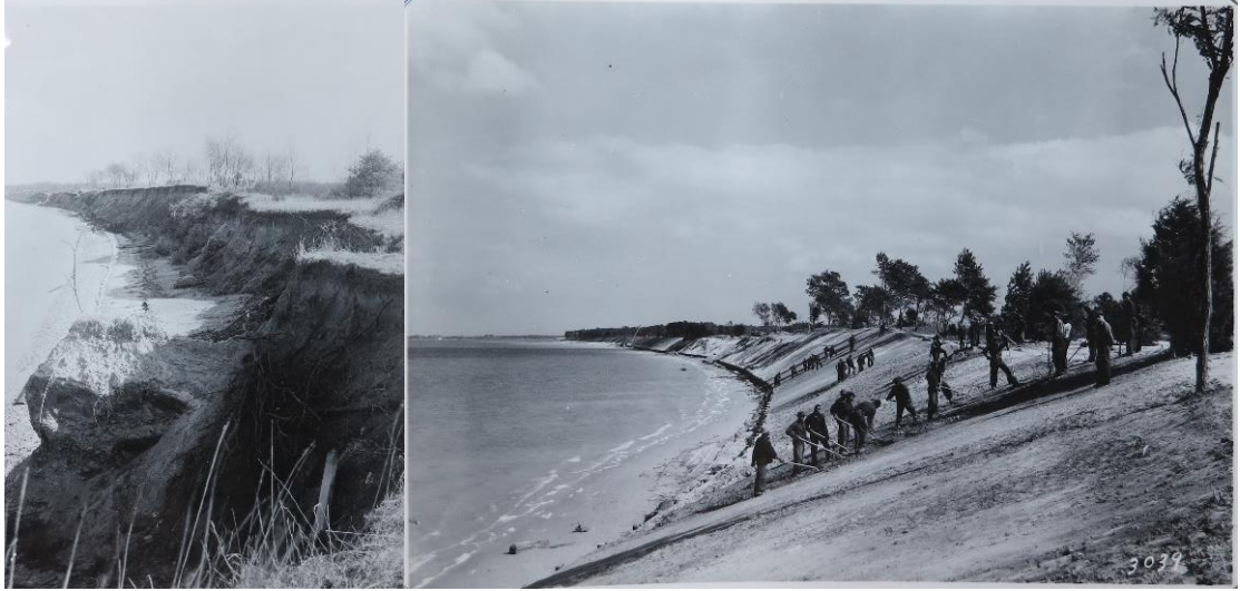
Figure 3. shoreline of Colonial National Monument both before (left) and after (right) CCC crews graded the area. 91
