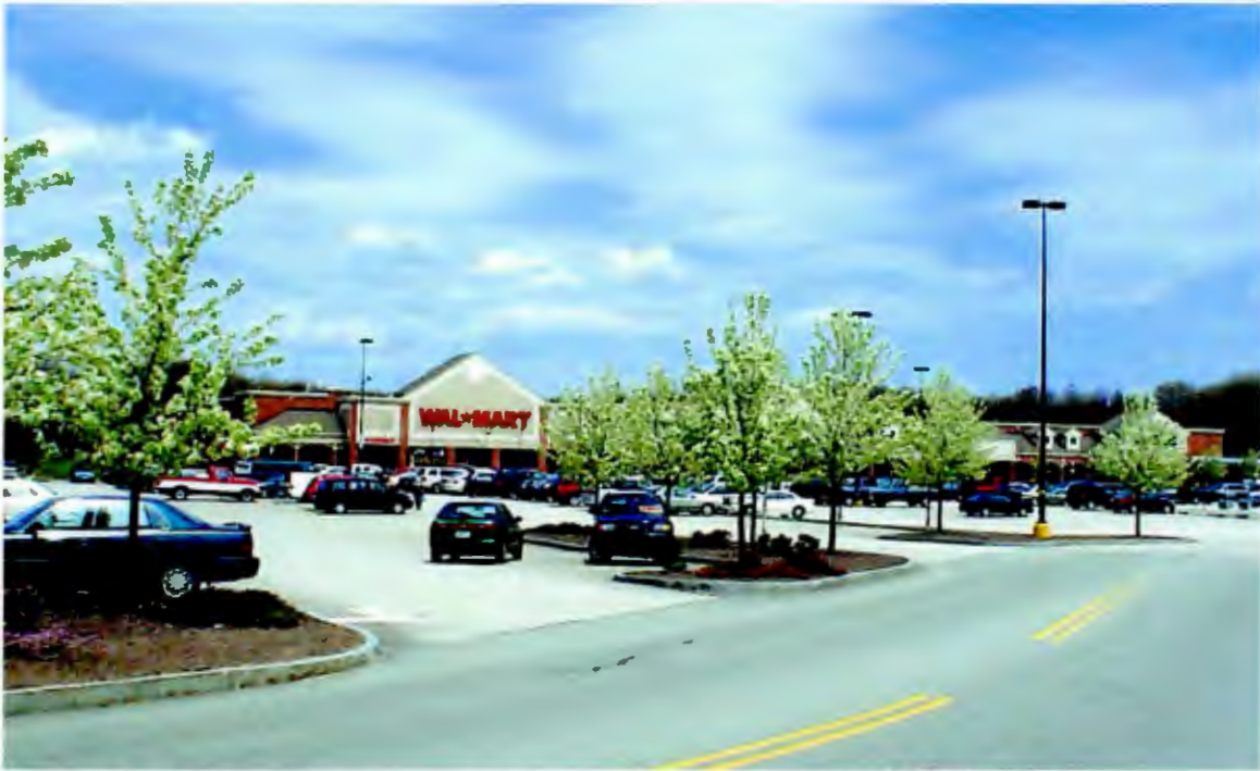
Figure 3.3. Wal-Mart with pitched roofs and additional landscaping. North Kingstown, RI.
