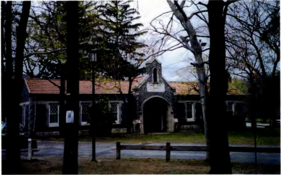
Figure 19.0 Main Gate House
