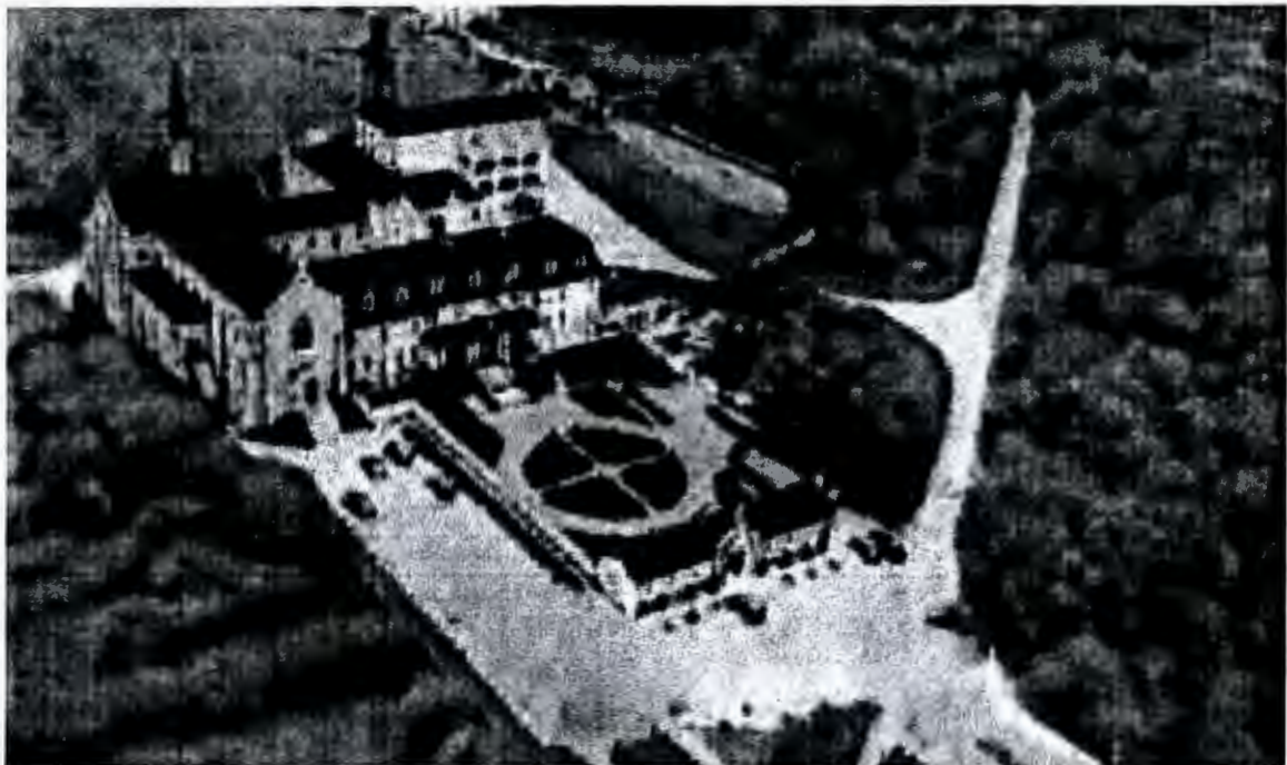
Figure 3.0 Aerial Photograph of the Monastery
