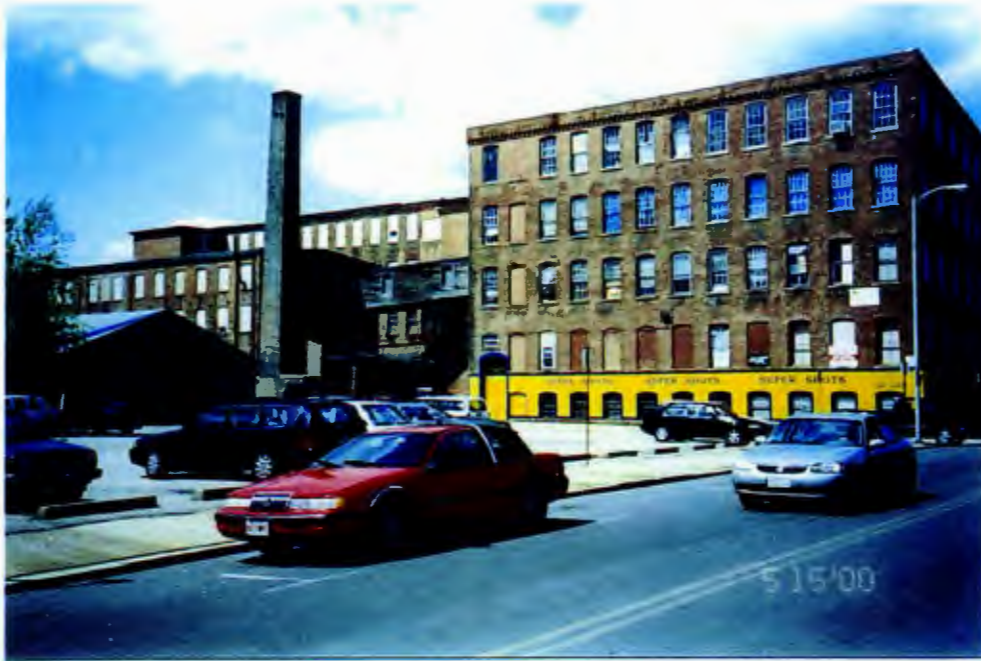
Figure 46: The Foster Building is an Example of an Underutilized Relic of Attleboro's Industrial Past
