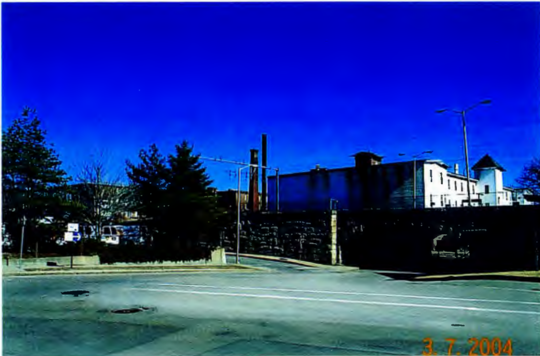
Figure 27: The MBTA Right-of Way at Mill Street
