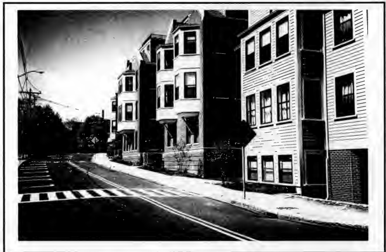
Kent Street at the Brookline Village Lofts.
