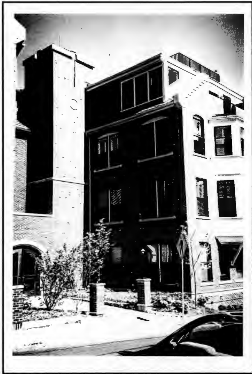
Brookline Village Lofts, elevator and entry at Building C
