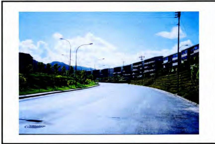
Figure 45. Interior road at Ciudad Casarapa.
