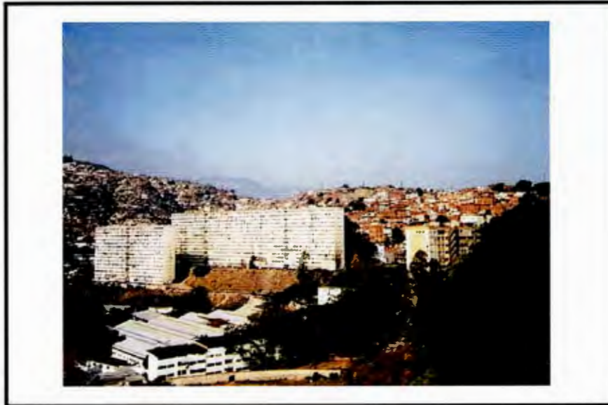
Figure 26. Public Housing and Barrios. © Fleming Bell, 1993.
