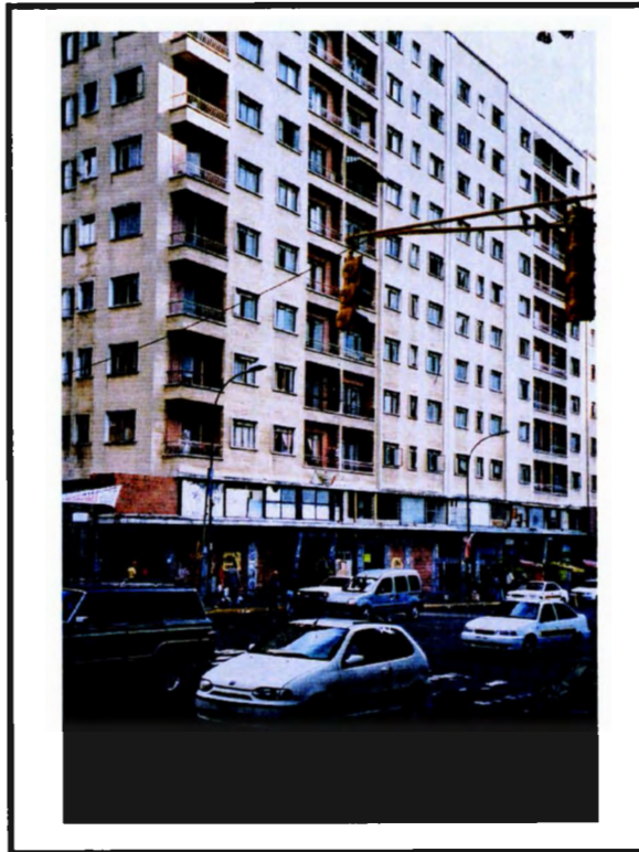
Figure 32. Vacant building, apparently under rehabilitation, at the west end of the Francisco Solano Ave. in the Parroquia El Recreo.
