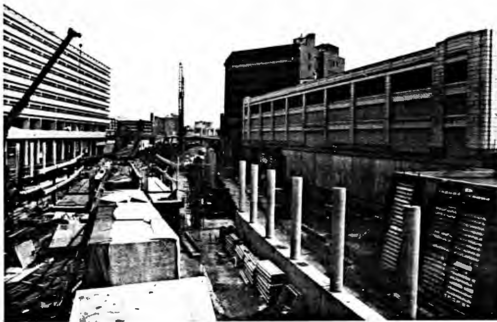
SOUTHWEST CORRIDOR (UNDER CONSTRUCTION)
