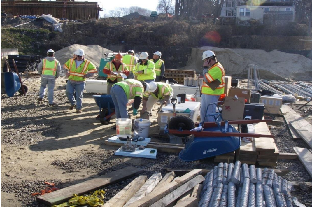
Figure 21 RIDOT and ATC testing personnel performing test on a concrete mix
