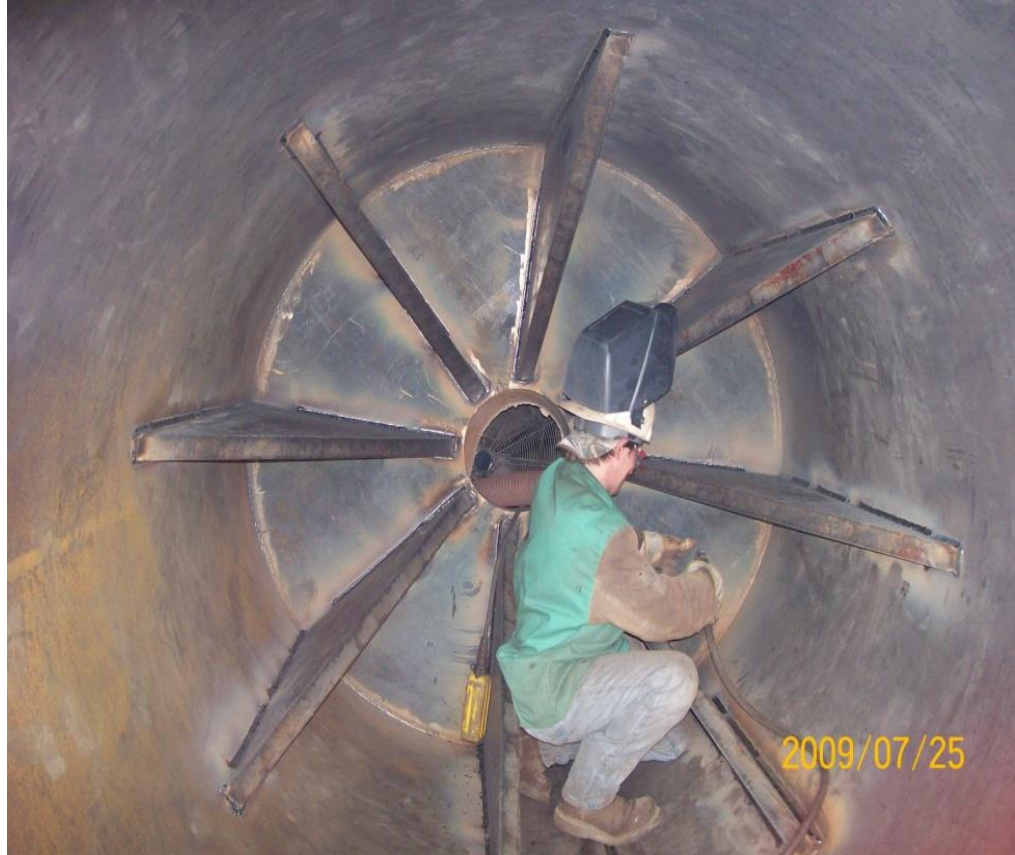
Figure 19 End Bearing Steel Plate
