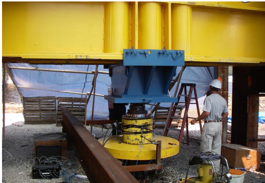
Figure 18 Load test on 48-inch steel pipe pile
