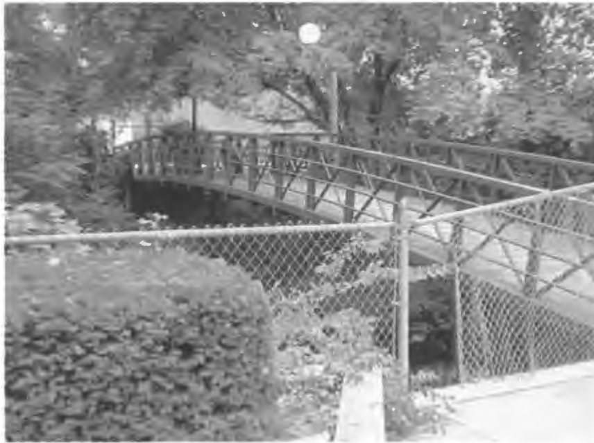
Figure 50: Pedestrian bridge over the Mill River
