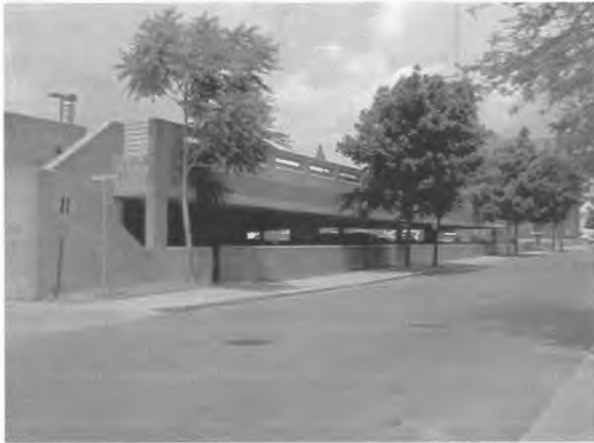
Figure 19: Municipal Parking Deck as Seen From Street
