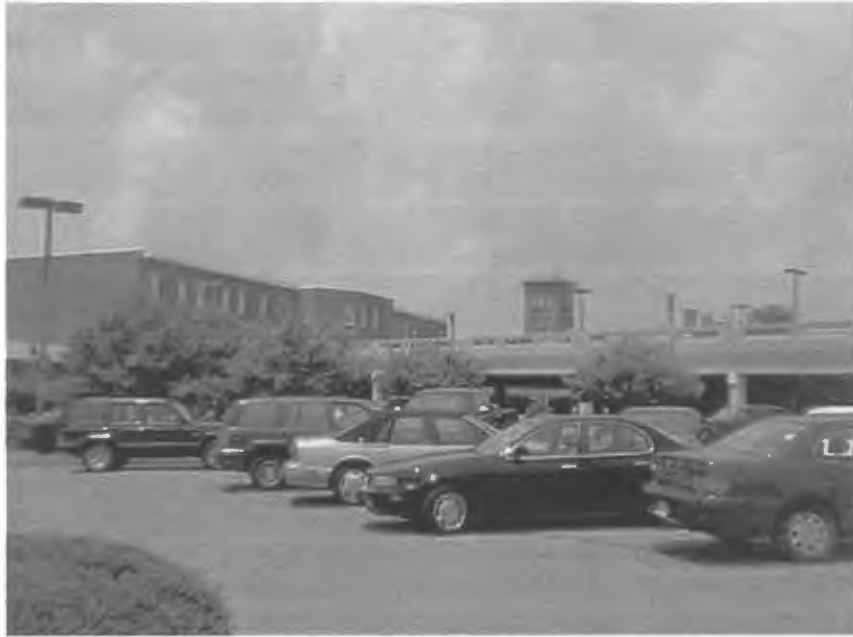
Figure 21: Parking Lot abutting the Municipal Parking Deck
