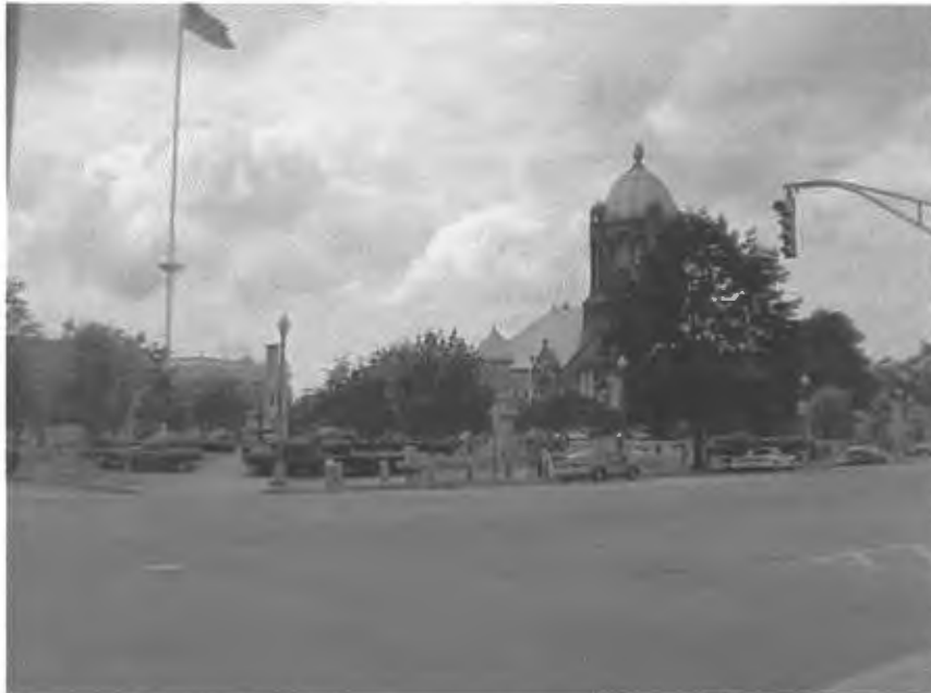
Figure 43: Taunton Green as seen from south side
