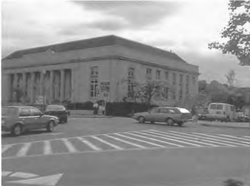
Figure 70 Court Street/ Taunton Green Intersection
