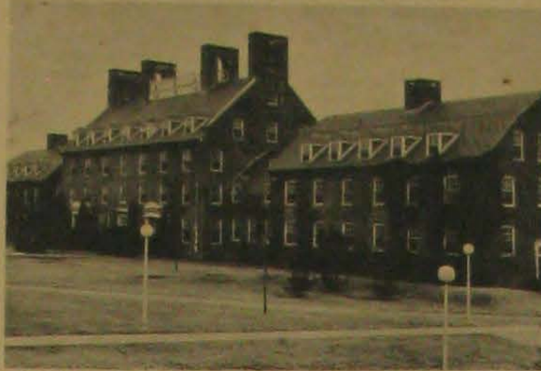
ROOSEVELT HALL , first dormitory built to house URI women in 1937, has been classified a fire hazard by state authorities.
