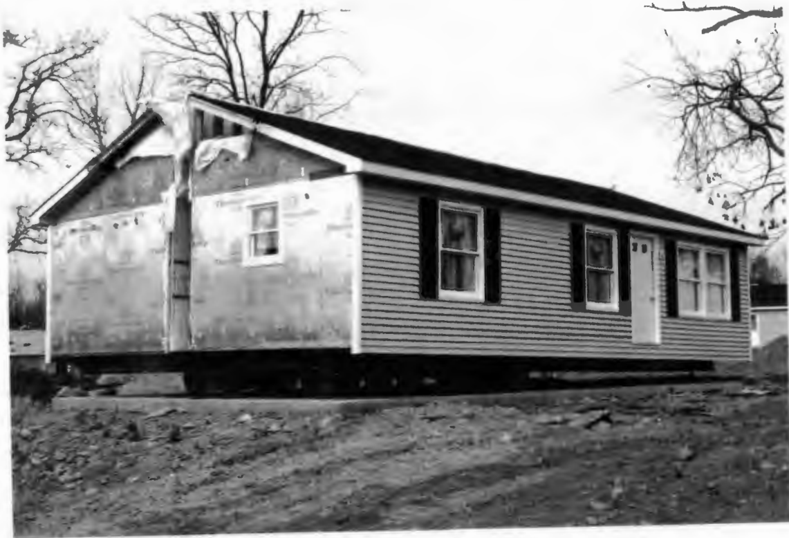
Each Half is Rolled Directly onto a Slab
