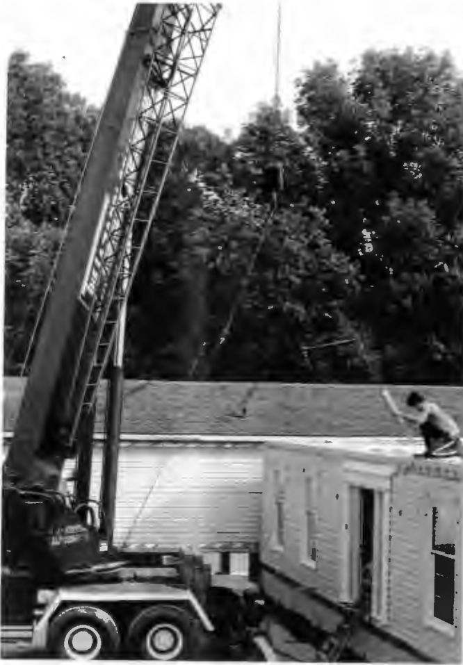
Crane Lifting a Module
