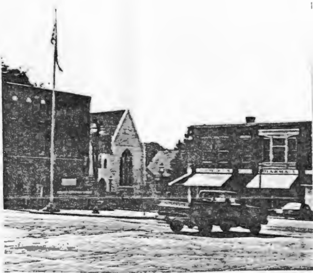
Traffic island is confusing and improperly designed.
