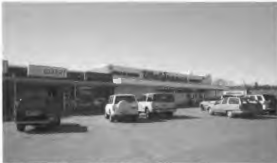
Figure 4.11 Walgreens in a former grocery store. 413 Washington Street, Stoughton, MA.
