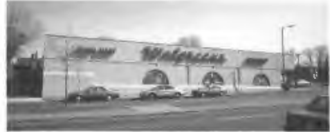
Figure 6.7 Community artwork on building elevation. 416 Warren Street, Roxbury, Massachusetts.
