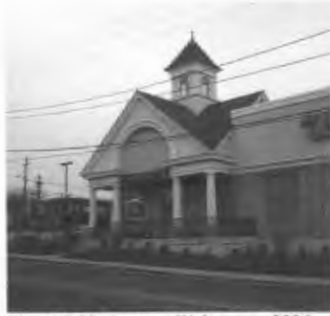
Figure 7.25 Access. Walgreens. 3336 Post Road, Warwick, Rhode Island.
