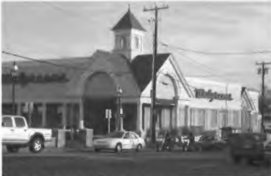
Figure 6.12 3336 Post Road, Warwick, Rhode Island.
