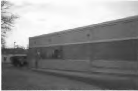
Figure 7.27 East elevation. Walgreens. 3336 Post Road, Warwick, Rhode Island.
