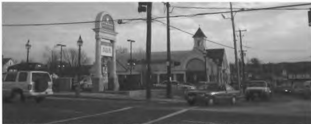
Figure 6.11 Retaining walls at corner of intersection. 3336 Post Road, Warwick, Rhode Island.
