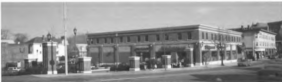
Figure 7.1 Walgreens, Corner of Harvard and Aspinwall Streets, Brookline, Massachusetts.
