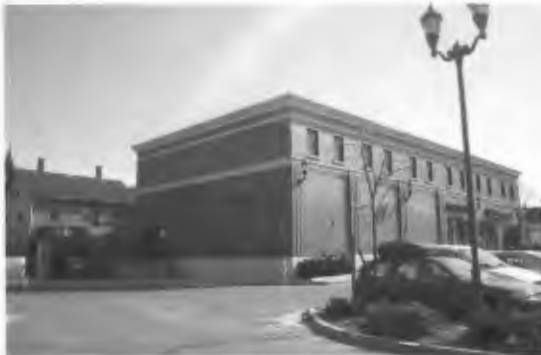
Figure 7.4 Rear Elevations. Walgreens, Brookline, Massachusetts.
