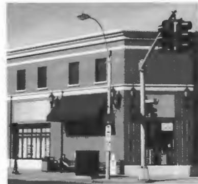
Figure 7.6 Bus Stop. Walgreens, Brookline, Massachusetts.
