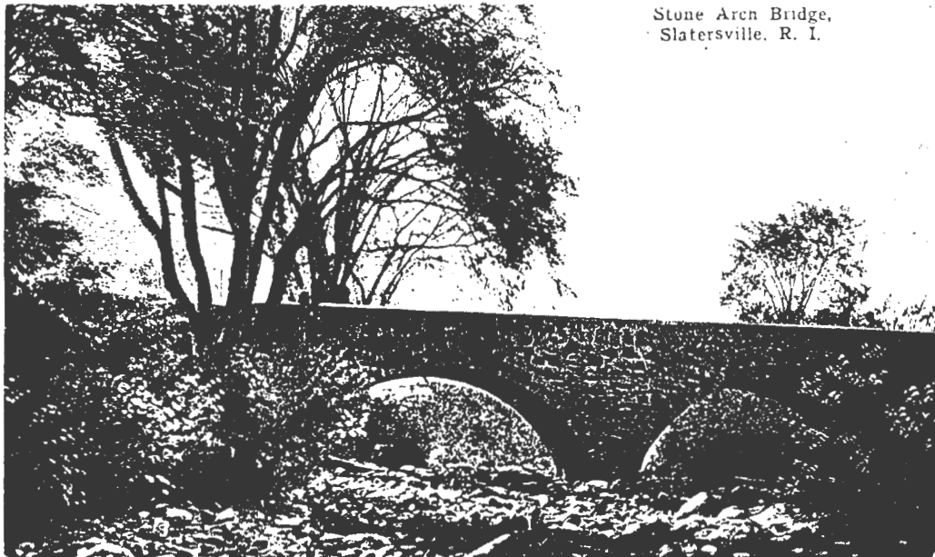
Figure 2.4 Stone Arch Bridge
