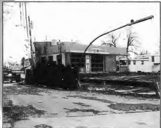
The underground gasoline tanks at this service station leaked into the ground and Narragansett Bay.
