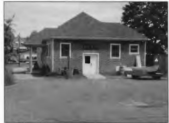
The Aspray Boat House serves as a community focal point. It is used by community groups, as a polling station and a meeting and resource area. Source: Gaspee Days Committee
