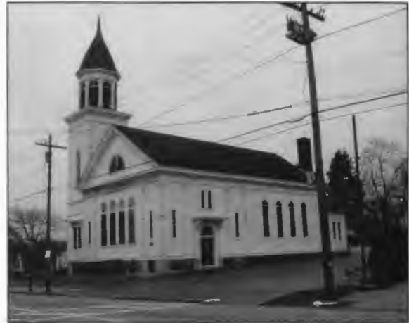
The historic Pawtuxet Baptist Church (1764) was covered in vinyl siding.
