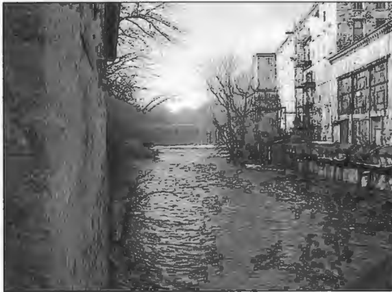
This is an abandoned textile mill on the Pawtuxet River. Source: Gaytha Langlois
