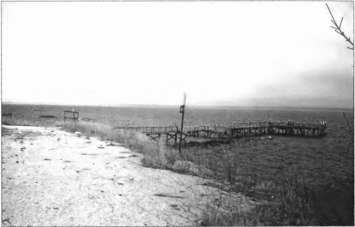
Figure 18. Rocky Point's Pier
