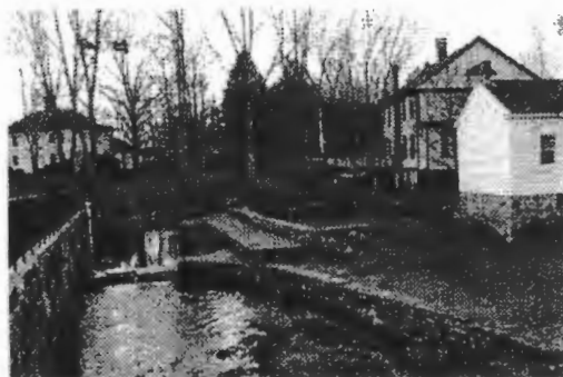
FIGURE 13: The stone retaining walls at the Shanuck River
