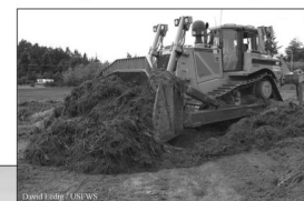
Salvage and relocation of top soil
