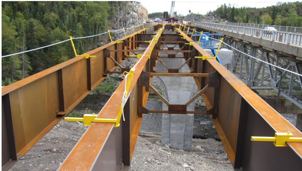
Figure 1.2: Typical I-shaped transversely stiffened steel plate girders (MRC, 2013).
