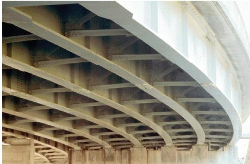
Figure 3.2.2: Typical short-span slab-girder steel highway bridge (Ryan et al., 2012).
