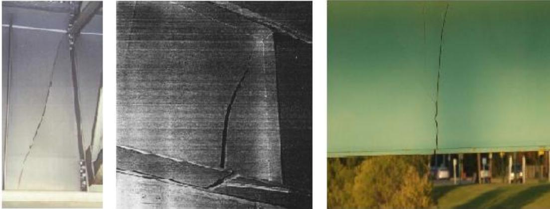
Figure 1.4: Fatigue-cracked steel plate girders (Kirke & Al-Jamel, 2004; Stockfish, 2011; Zhou & Biegalski, 2010).
