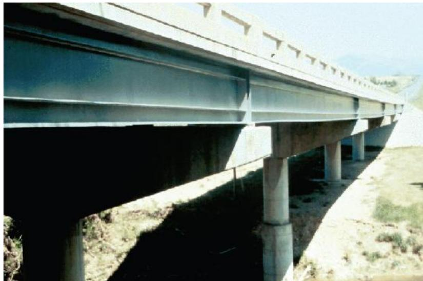
Figure 1.1: Typical short-span slab-girder steel highway bridge (Ryan, Mann, Chill, & Ott, 2012).
