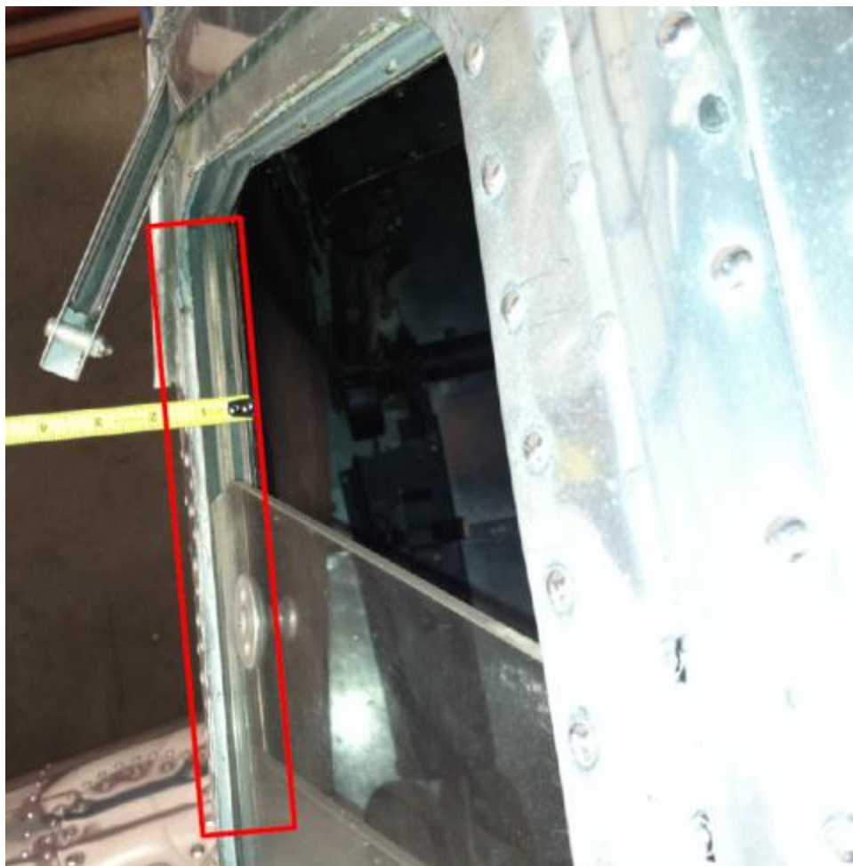
110 111 Figure 4: Parallel rails constrain the side window and allow it to slide.
