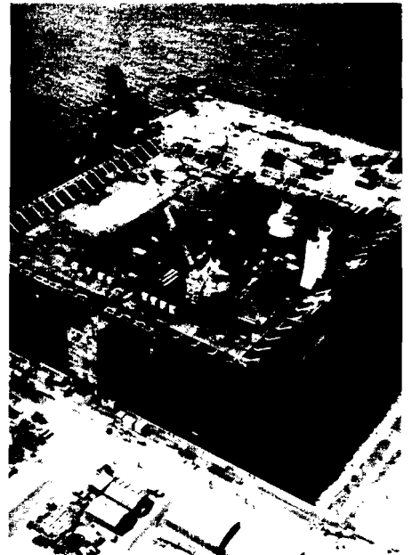
6. Assembly of the upper deck completed (October 1974)
