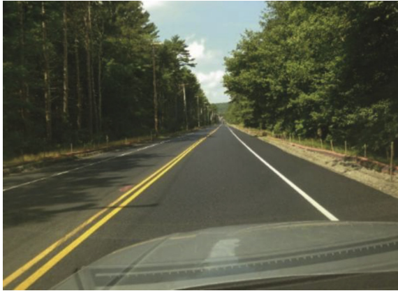
Fig. 4 – Route 165 view after rehabilitation in 2014.
