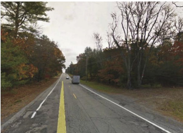
Fig. 1 – A view of Route 165 before rehabilitation in 2013.
