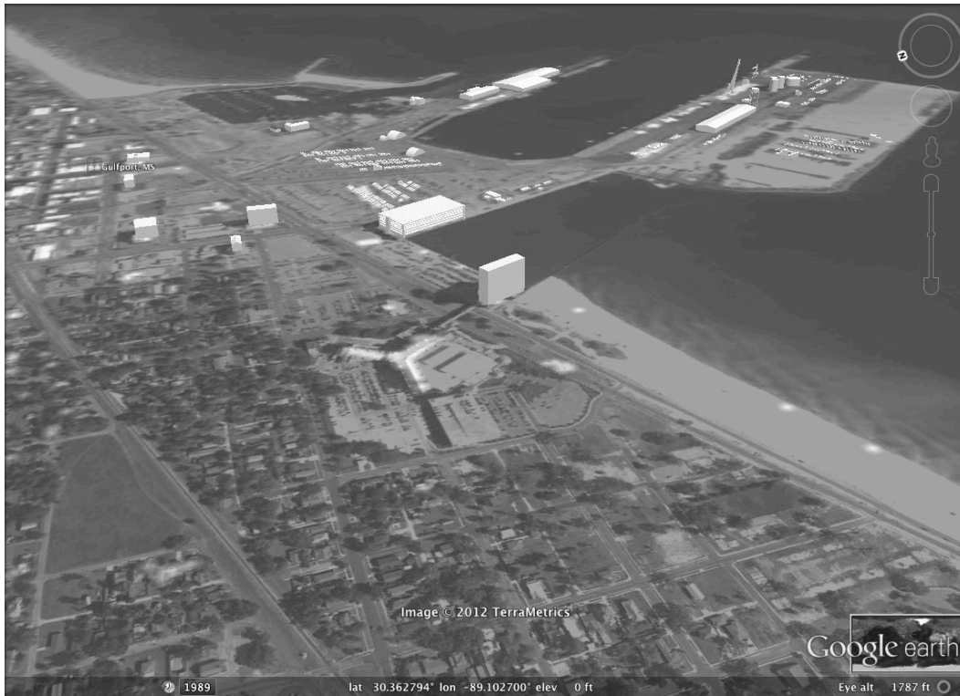
Figure 9 -- Port of Gulfport with simulated Category 4 storm surge
