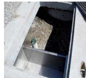
**Figure 8:** Interior of tree filter system ready for tree planting. In foreground, "pre-treatment" sump with weep holes; bypass/overflow pipe also shown.
